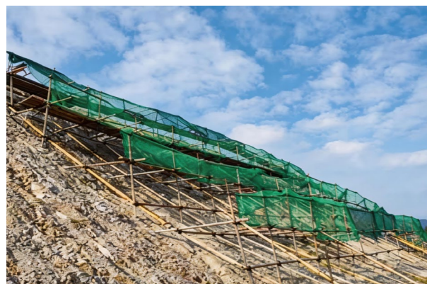
Slope Remediation at 1370-1358 Section, Woniuping Mine, Sichuan Ya Dong
