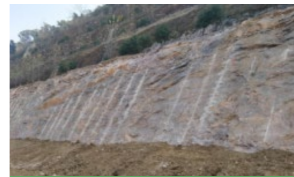
Jiangxi Ya Dong has implemented pre-split blasting on the final slopes of its mining area to ensure the integrity and stability of the rock mass.
