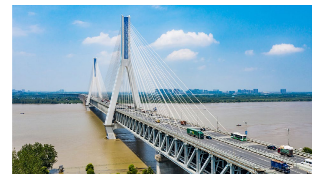
Tianxingzhou Yangtze River Bridge in Wuhan
