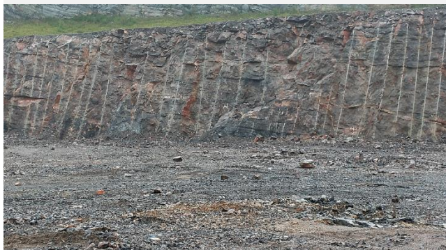
Pre - split blasting is carried out at the end of the slope to maintain the integrity and stability of the rock mass.
